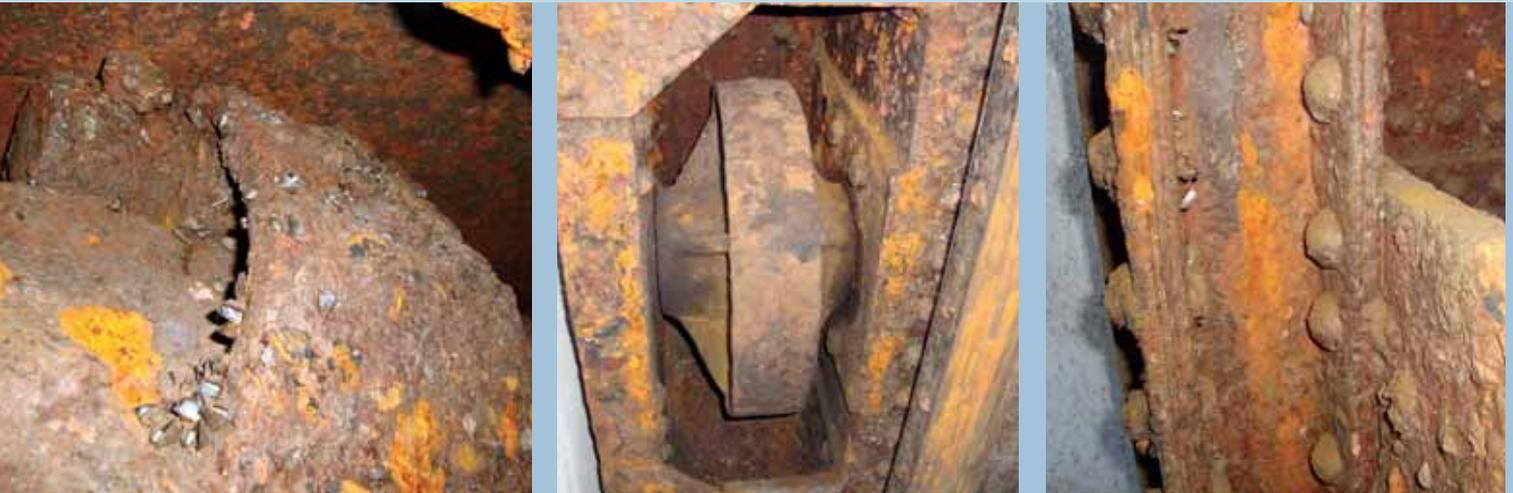
Severe plate rust and shell deposits on pumped-storage power plant components: fastening element, guide roller and rivet connection of section and sheet
